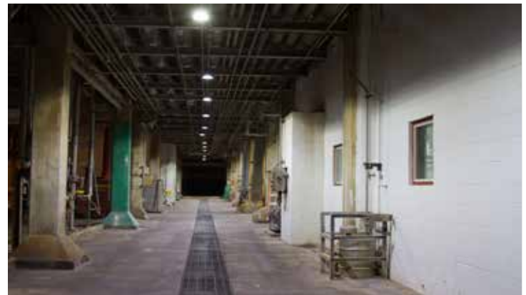
Dialight SafeSite LED High Bays increase visibility and safety in the facility.
